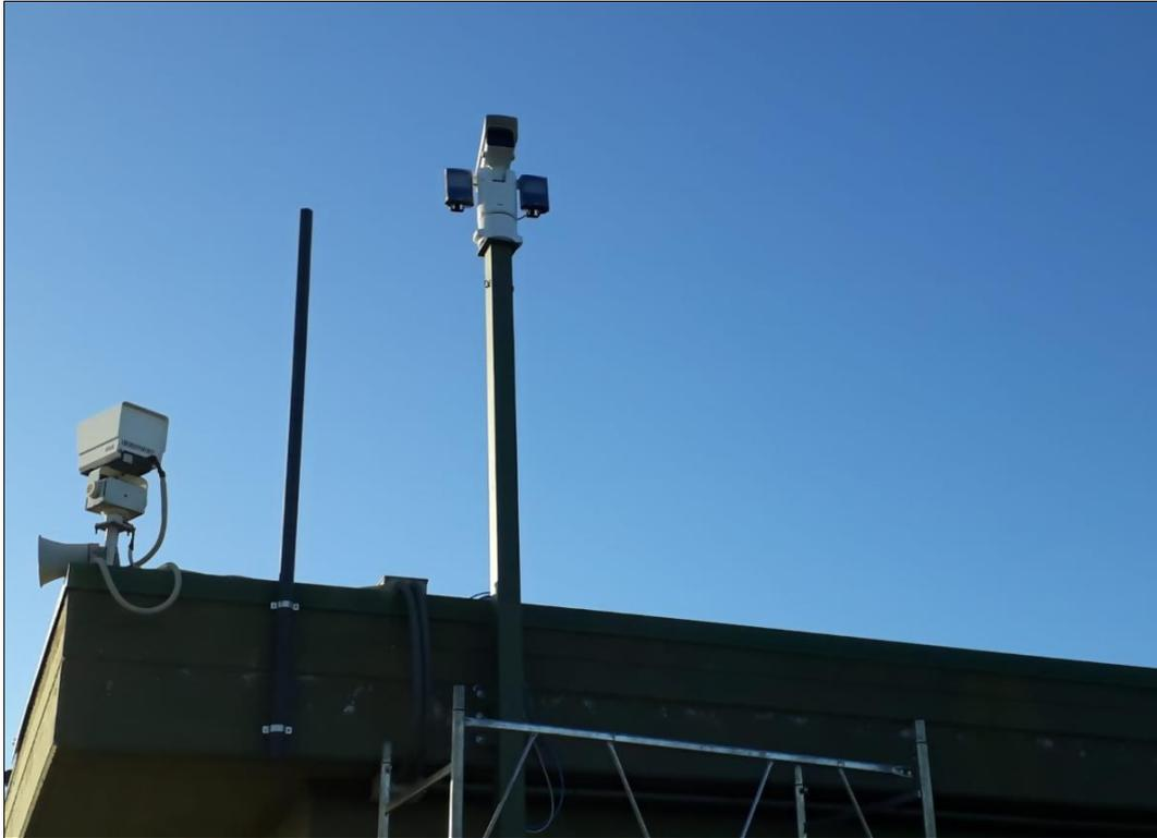
*Installation at the 4th Air Force Wing of Grosseto of intelligent cameras for bird-detection*
